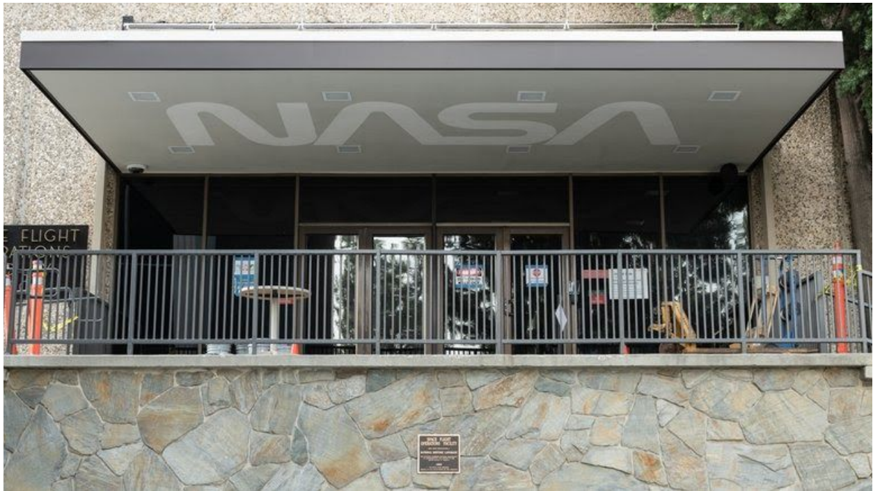
A NASA worm logo has been painted on the entrance overhang of Building 230.
