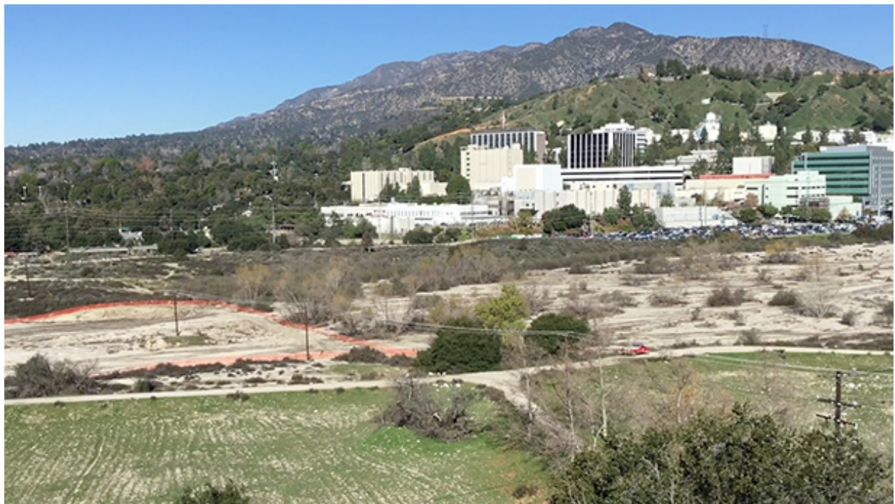
The Arroyo area south of JPL.
