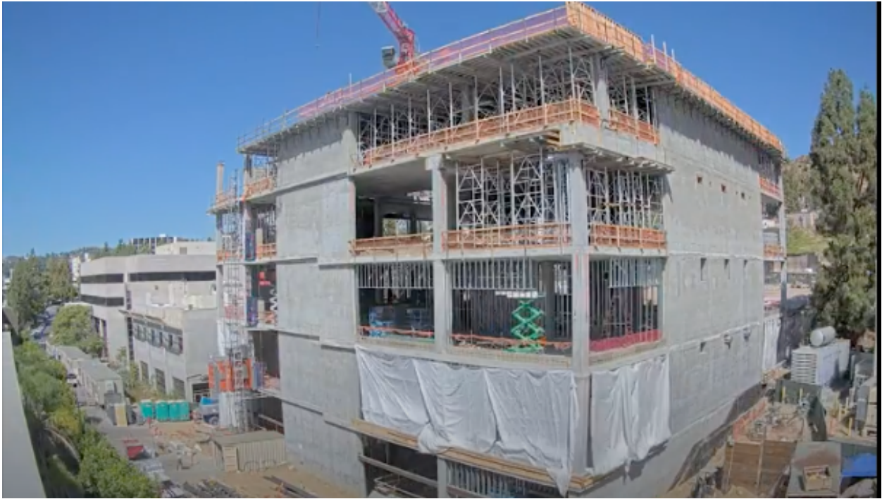
Building 350 under construction.
