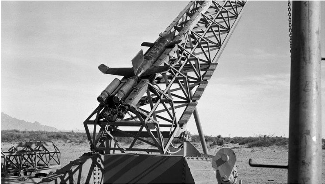
The Private F launcher tower, redesigned to accommodate the missile's wings.
