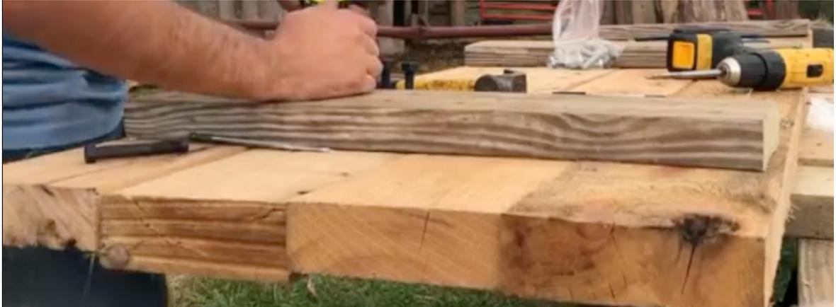
**Step 2** : Turn the platform upside down and use the spacers provided to drill 2 x holes at each corner of the platform. Space these holes and the load cells close to the edge of the platform.
